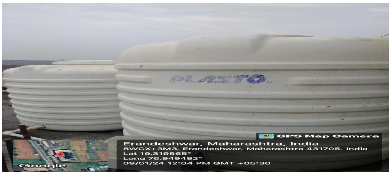
Water Harvesting tank (Capacity-1000L)
